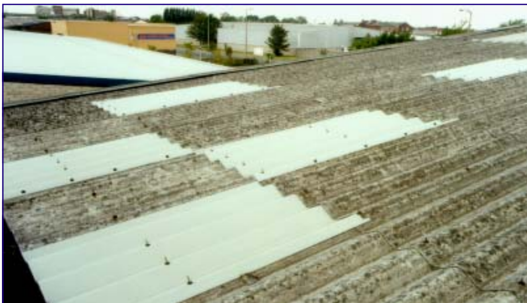
Doublesix M Profile FILON DR Used as a Direct Replacement for Asbestos Cement Sheeting
