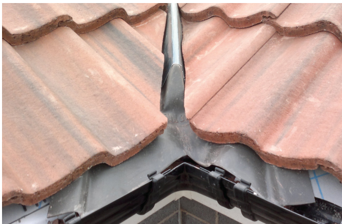
E. The eaves closure piece is cut to allow water discharge into the gutter.
